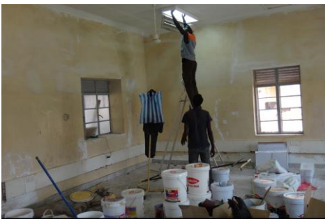
Repairing ceilings and painting the Pediatric Ward
