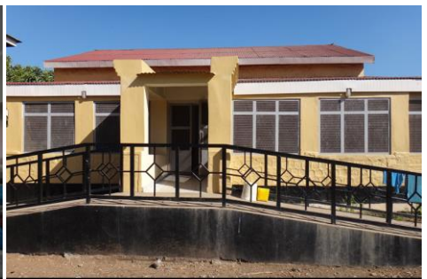
Entrance to Pediatric Ward after renovations
