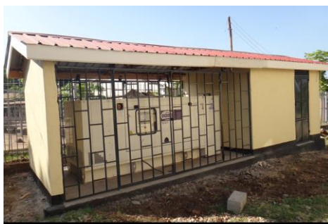
RMF built generator housing
