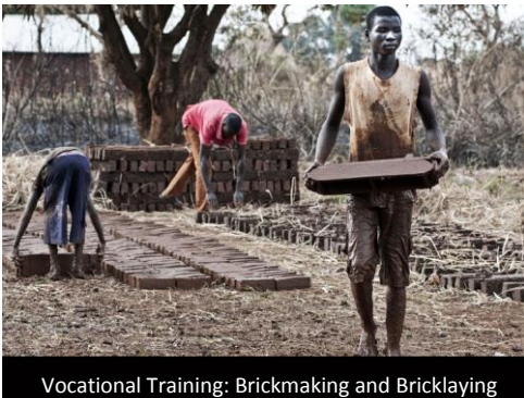
Vocational Training: Brickmaking and Bricklaying
