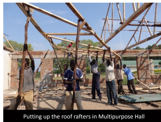
Construction begins in late 2013
